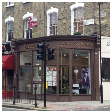
Photo 29: Locally listed building
