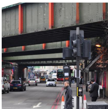
Photo 22: Seven Sisters Road viaducts
